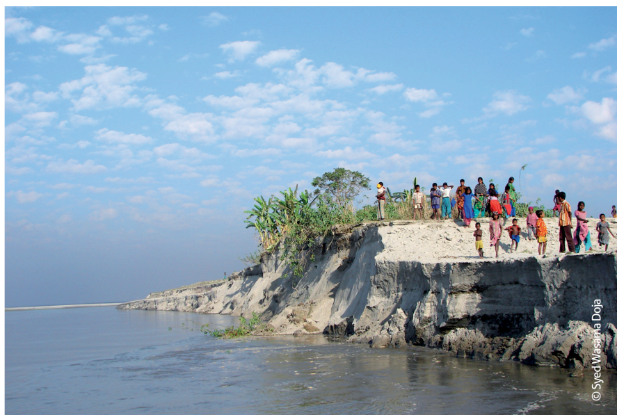
[1] Land erosion in Gaibandha district, Bangladesh.
